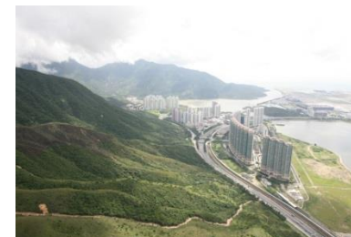
Slope monitoring site, Tung Chung, HK
